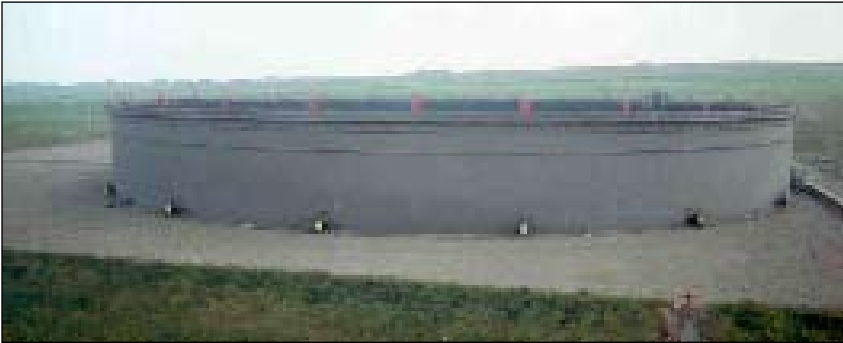
Plenty swivel angle belt drive mixers on a 1,000,000 Bbl (160,000 m 3 ) crude oil tank in Europe.
