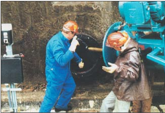
Installing a Plenty belt drive mixer in Europe
